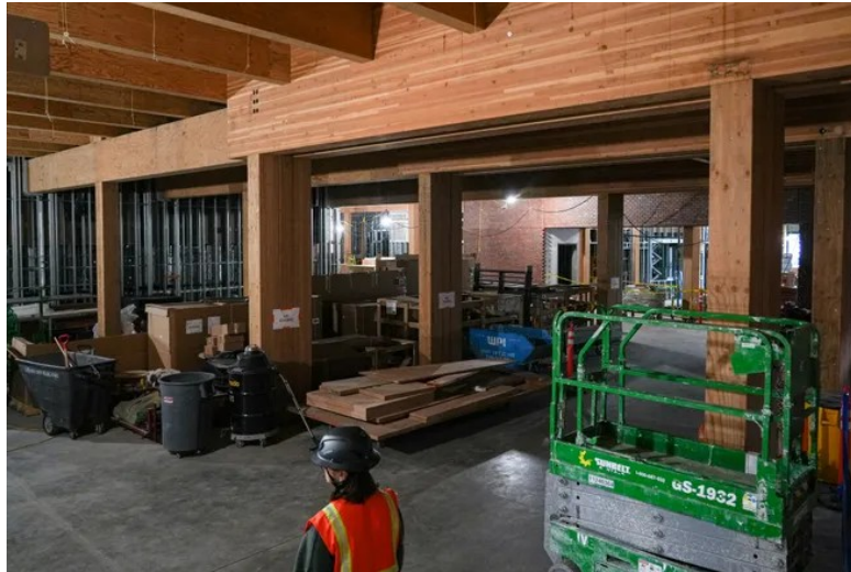
Figure 2: Inside the OSU Huang Complex, where the new data center and XRT space are being built.
